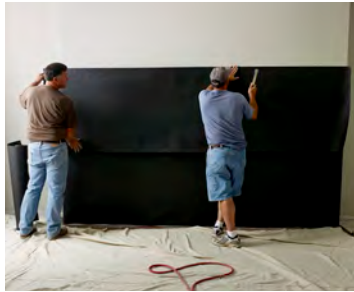
Install weather-resistant barrier.
