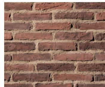
Overgrout Joint
