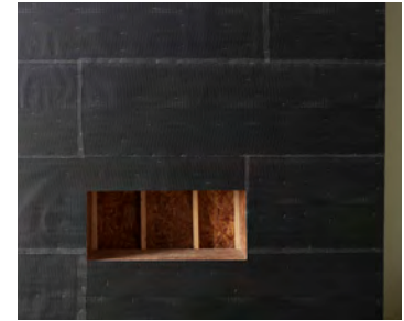
Wall ready for mortar scratch coat.
