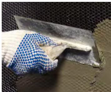
Cover entire lath with mortar.
