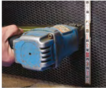
Attach lath to weather-resistant barrier.
