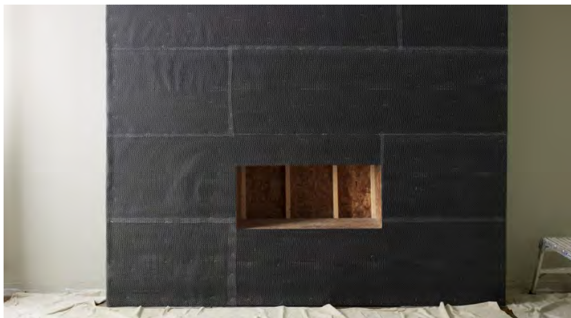
Chalk lines assist to keep joints straight.
