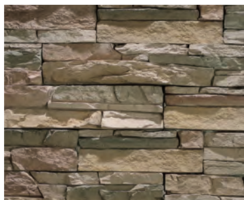
Dry-stack Joint
